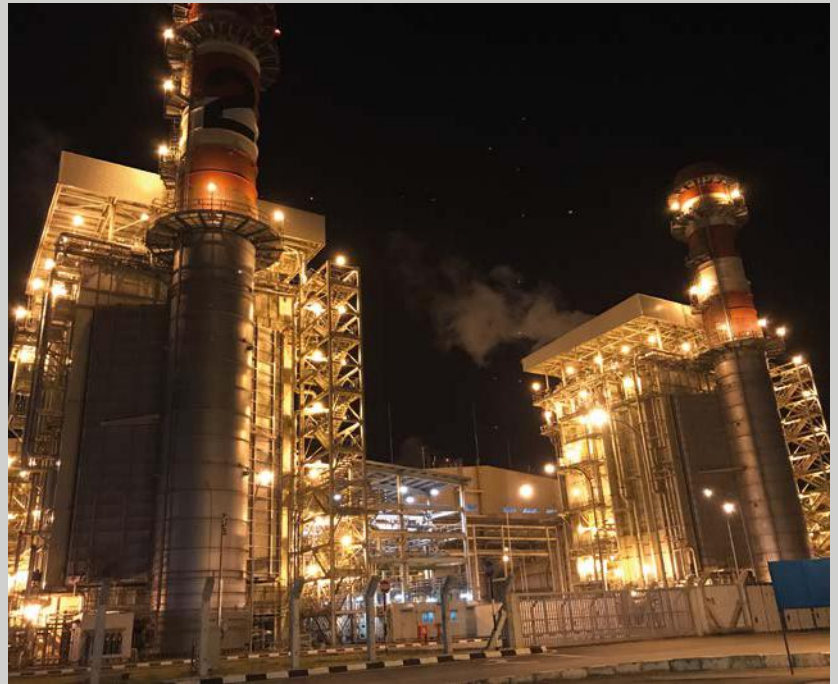
Combined Cycle Power Plant (CCPP) in Pray, Malaysia (at night)
