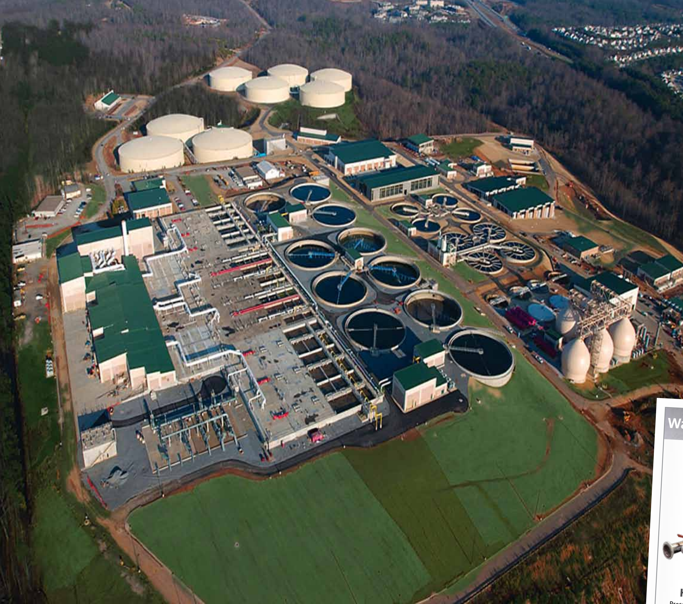
Ft. Wayne Hill Treatment Facility, Gwinnett County, GA
