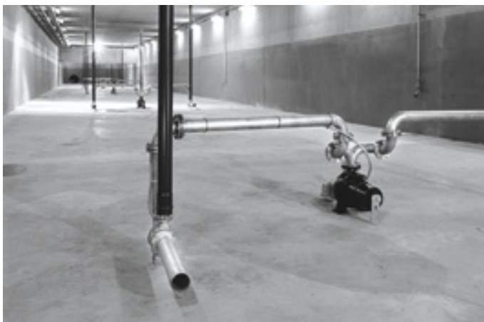
A stormwater and sewage retention tank with a capacity of 22,500 m 3 and a floor area of 4,300 m 2 . 24 KSB Amajets, total power 384 kW.
